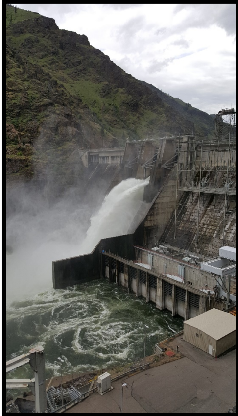
FIGURE 4 OXBOW DAM IN OPERATION MAY 22, 2019
